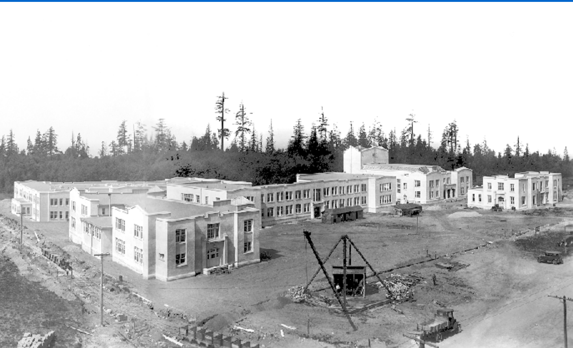
Construction of “Semi-Permanent” Buildings and Power House (1925)
