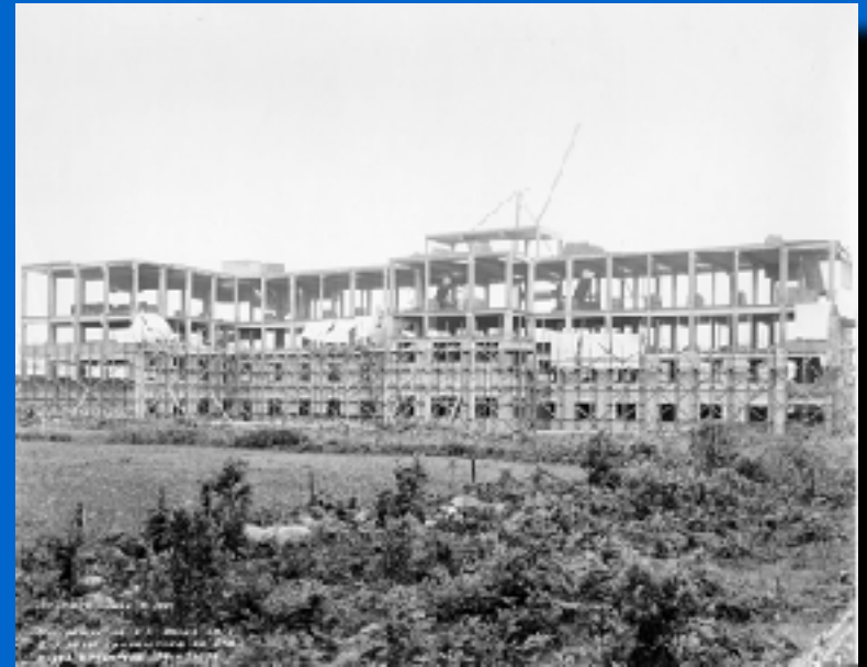
Science Building under construction (1923)
